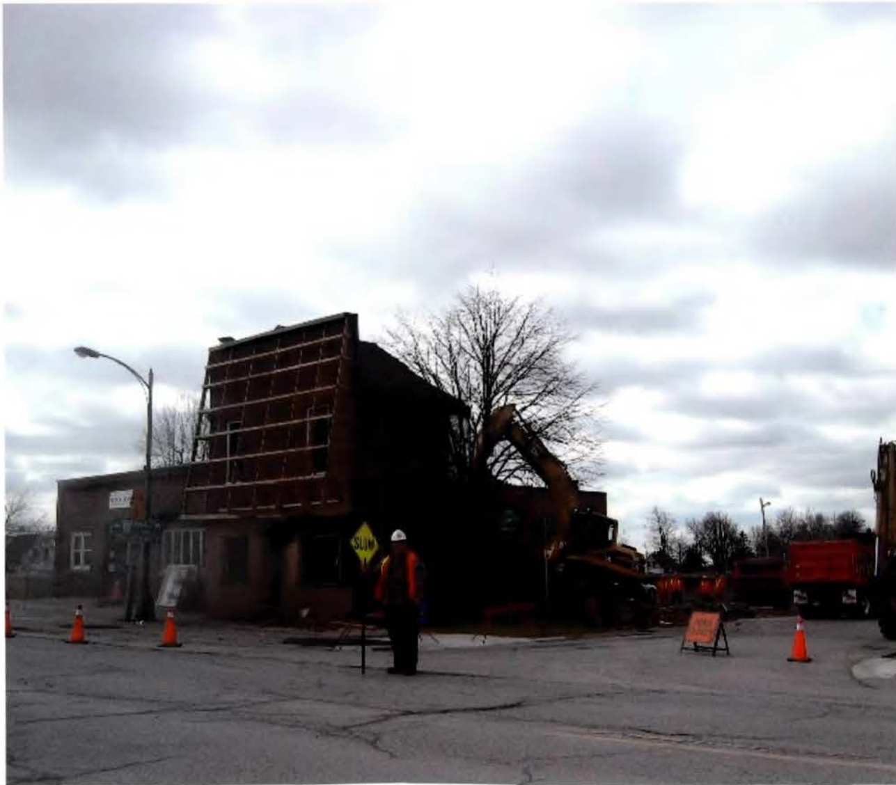
The Dutton Advance under demolition. April 2007.
